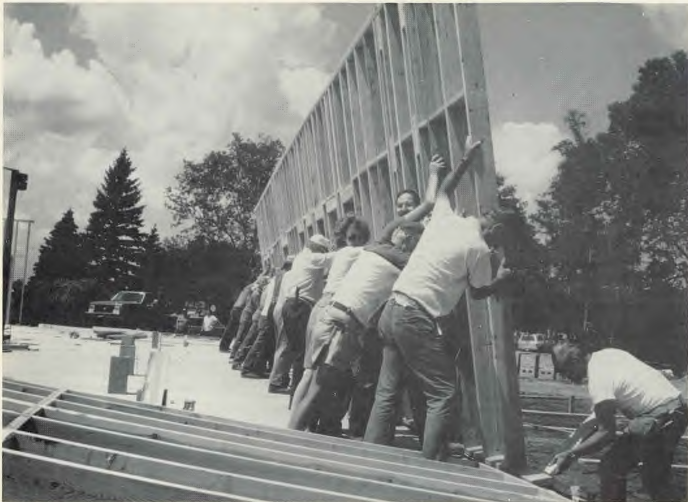
One, two, three and up with a wall on the Pipestone church. It was teamwork—Maranatha volunteers, church members, Conference personnel, and friends working together that built the Pipestone church.
