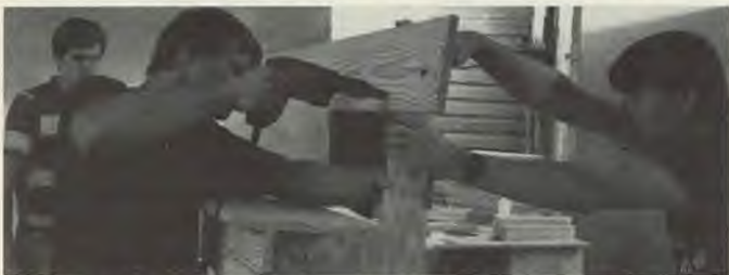
Twenty 12-foot-long pews were built for the church. Pictured are Don Salt, music teacher at Maplewood; Dave Zilmer from Karlstad and Pastor Ken Mayberry from Karlstad.
