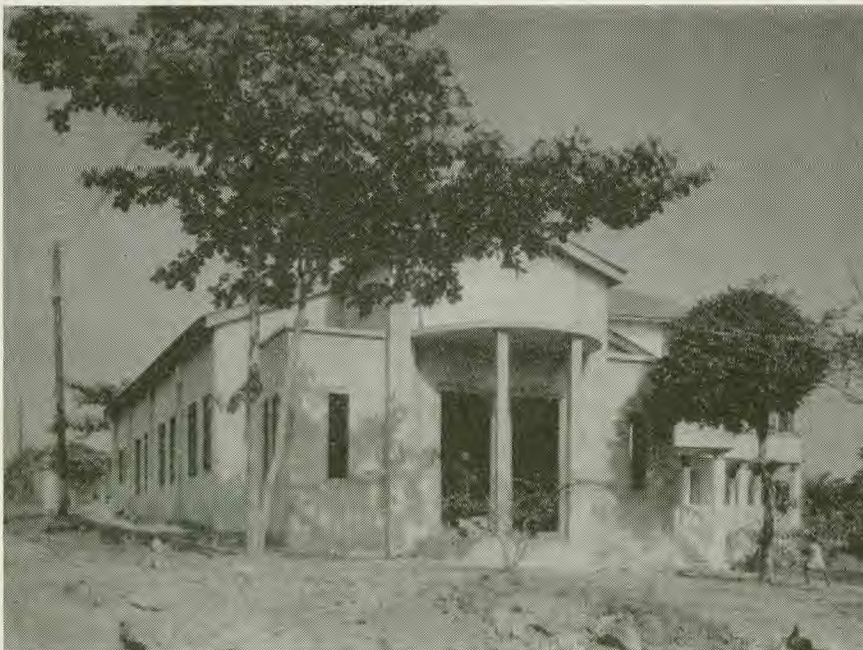
Church Building in Monrovia, Liberia, Nearing Completion. Seating Capacity 250
