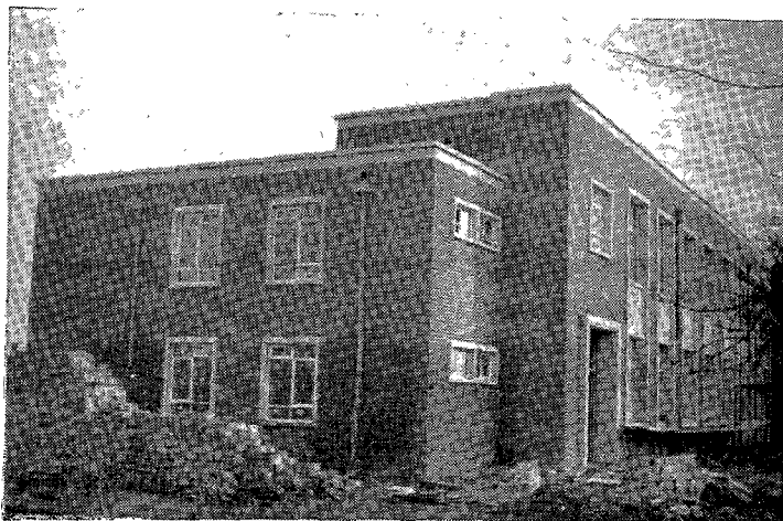
Portion of the new Administrative Building at Newbold College makes rapid progress toward completion.
