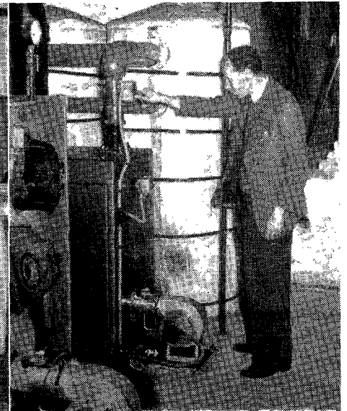
David R. Throssell, Maintenance Engineer of the College, is here seen adjusting the controls on the recently installed Moor Close boiler.
