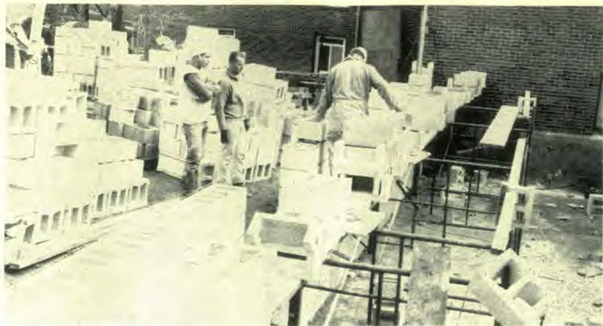
Walls of the dormitory addition at UCA are going up.
