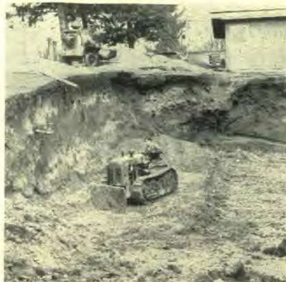
Excavation for the dormitory and dean's quarters addition at UCA.
