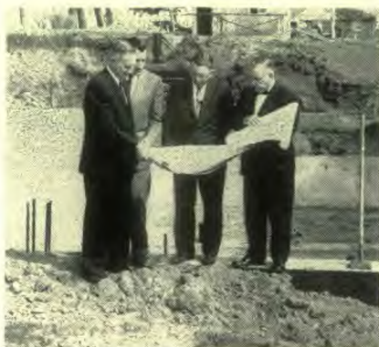
(Left to right) Principal F. E. Schlehuger, Academy Treasurer W. H. Dick, Conference Treasurer W. E. Wasenmiller, and President C. M. Bunker study building plans on the site of new construction at UCA.
