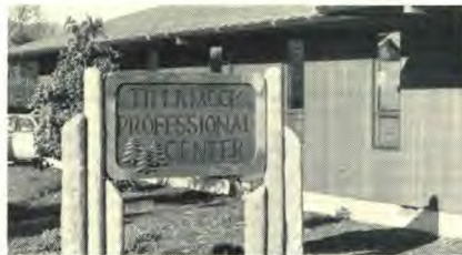
Tillamook Professional Center is located adjacent to Tillamook County General Hospital and facilitates the meeting of healthcare needs for Tillamook and the surrounding county.
