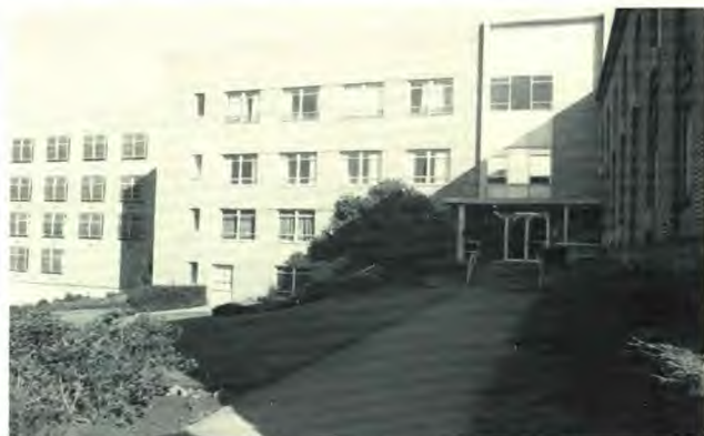
The convalescent center uses this newest wing of the former Portland Adventist Hospital on Mt. Tabor.
