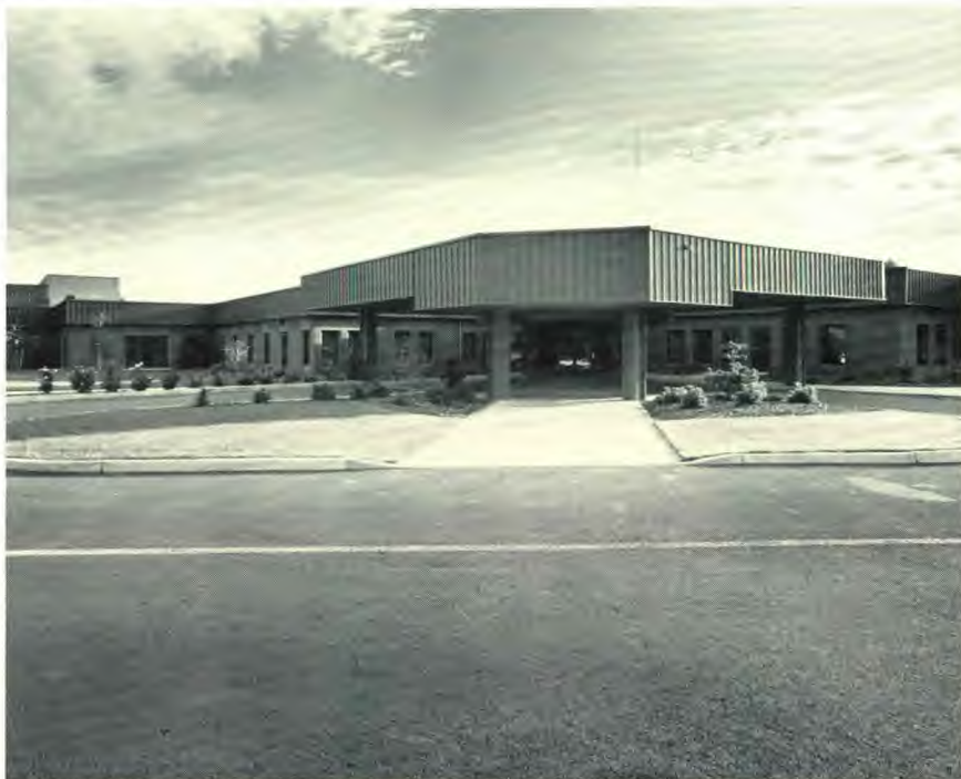
The main entrance of the new Walla Walla General Hospital.
