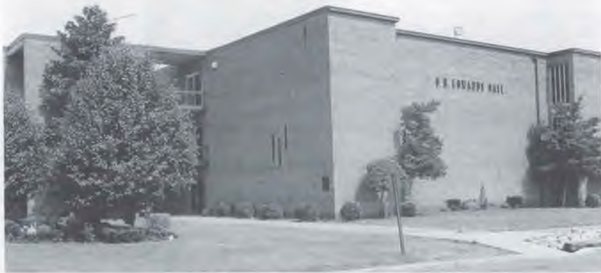
The 1987 Oakwood College offering helped remodel Edwards Hall, the men's residence.
