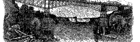
MICHIGAN CENTRAL NEW CANTILEVER BRIDGE, NIAGARA FALLS.
