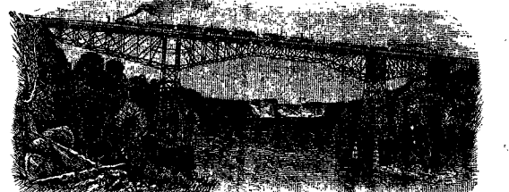
MICHIGAN CENTRAL NEW CANTILEVER BRIDGE, NIAGARA FALLS.
