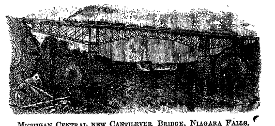
MICHIGAN CENTRAL NEW CANTILEVER BRIDGE, NIAGARA FALLS.
