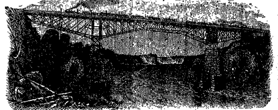
MICHIGAN CENTRAL NEW CANTILEVER BRIDGE, NIAGARA FALLS.
