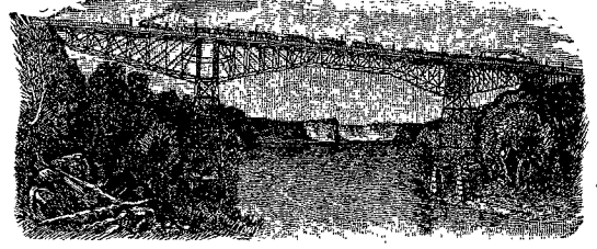
MICHIGAN CENTRAL NEW CANFIELDER BRIDGE, NIAGARA FALLS.
