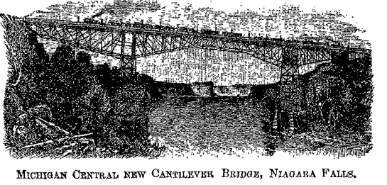
MICHIGAN CENTRAL NEW CANTILEVER BRIDGE, NIAGARA FALLS.
