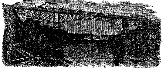
MICHIGAN CENTRAL NEW CANTILEVER BRIDGE, NIAGARA FALLS.
