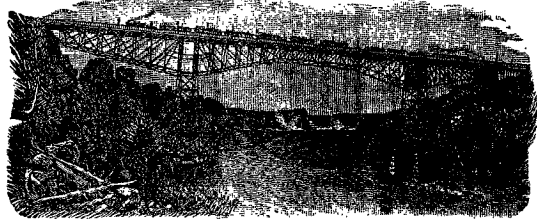
MICHIGAN CENTRAL NEW CANTILEVER BRIDGE, NIAGARA FALLS.
