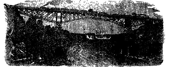
MICHIGAN CENTRAL NEW CANTILEVER BRIDGE, NIAGARA FALLS.
