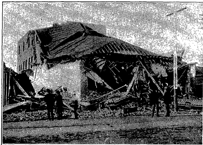
ONE OF THE WRECKED BUILDINGS IN HEALDSBURG
