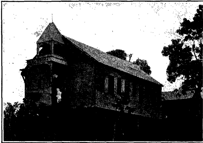
CHURCH (NEARING COMPLETION) AT MT. HOPE, CANAL ZONE.
