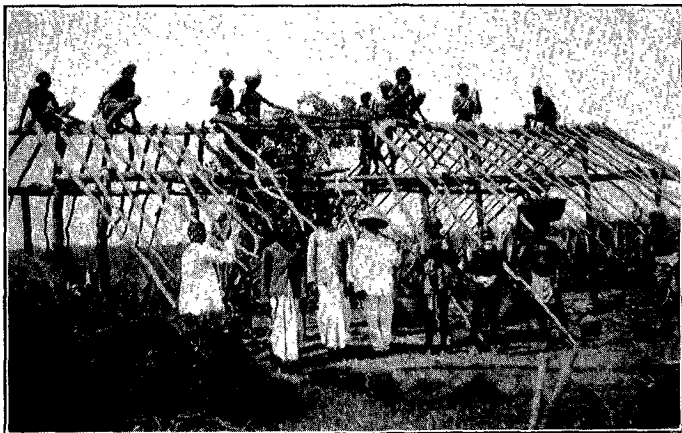
SANTALS BUILDING CATTLE-SHEDS ON BABUMOHAL MISSION
