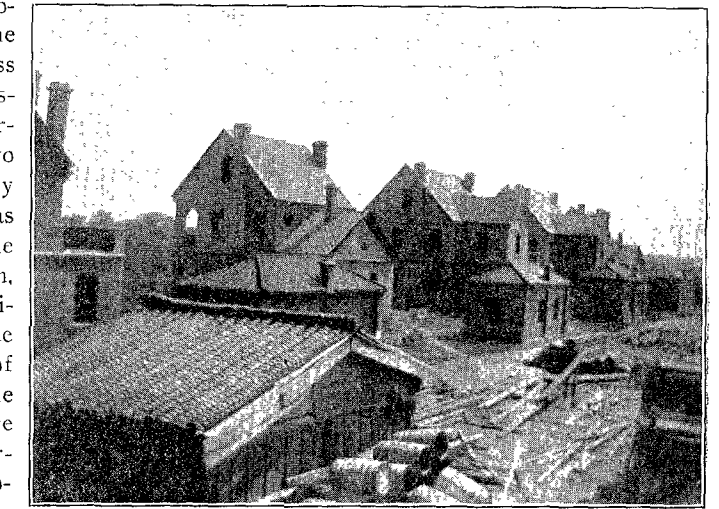
REAR VIEW OF HOMES FOR FOREIGN WORKERS IN SHANGHAI, CHINA
