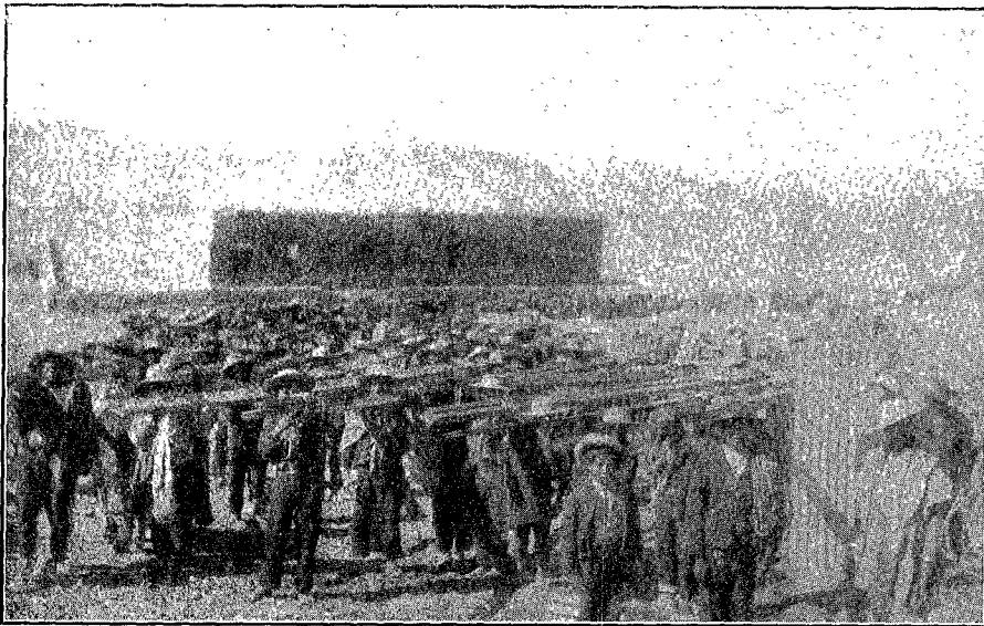
INDIANS BRINGING MATERIAL FROM PUNO, TWENTY-ONE MILES, UPON THEIR SHOULDERS FOR THE NEW MISSION BUILDING
