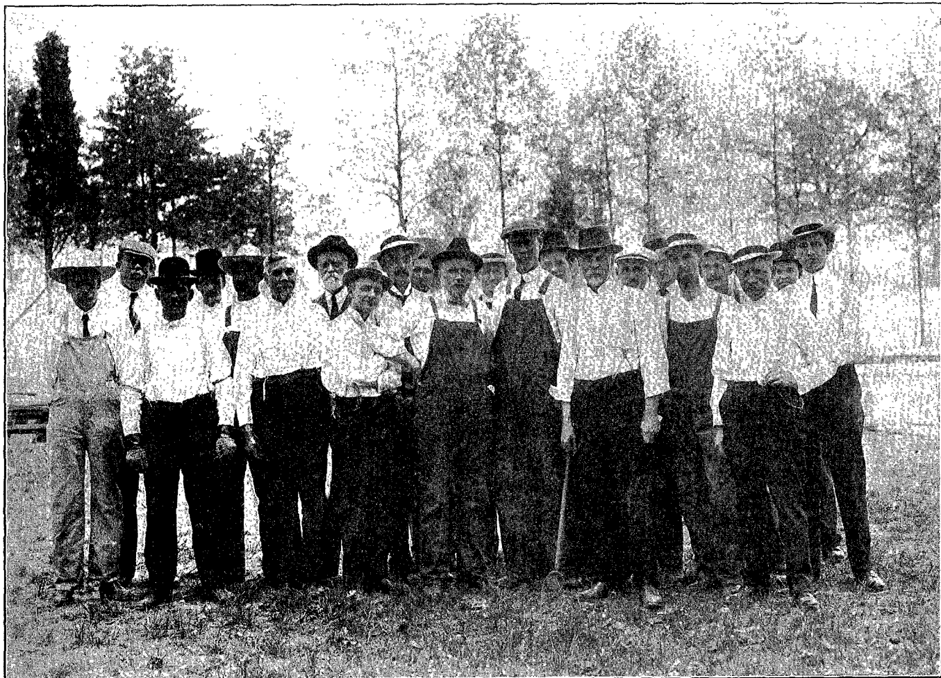
A FEW OF THE CAMP-CONSTRUCTION WORKERS AT THE GENERAL CONFERENCE, PREPARING TO LIFT THE POLES FOR THE LARGE PAVILION
