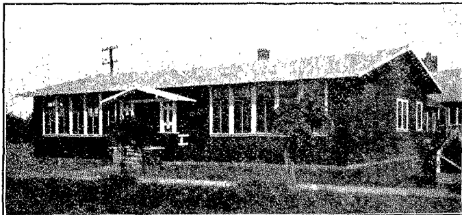
MOUNTAIN VIEW (CAL.) CHURCH SCHOOL BUILDING
