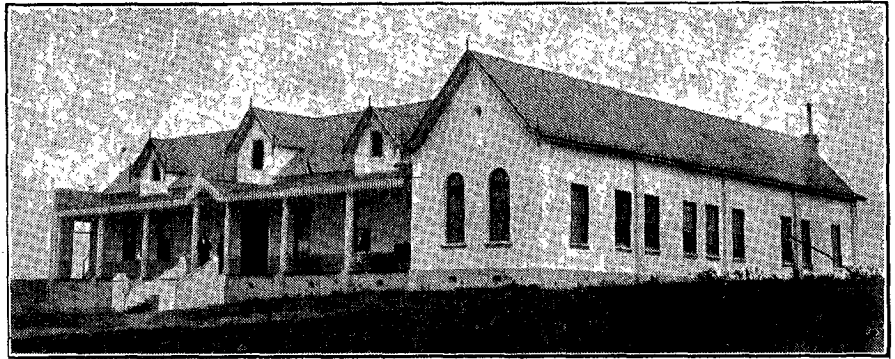
MAIN BUILDING OF SAO PAULO, BRAZIL, SCHOOL
