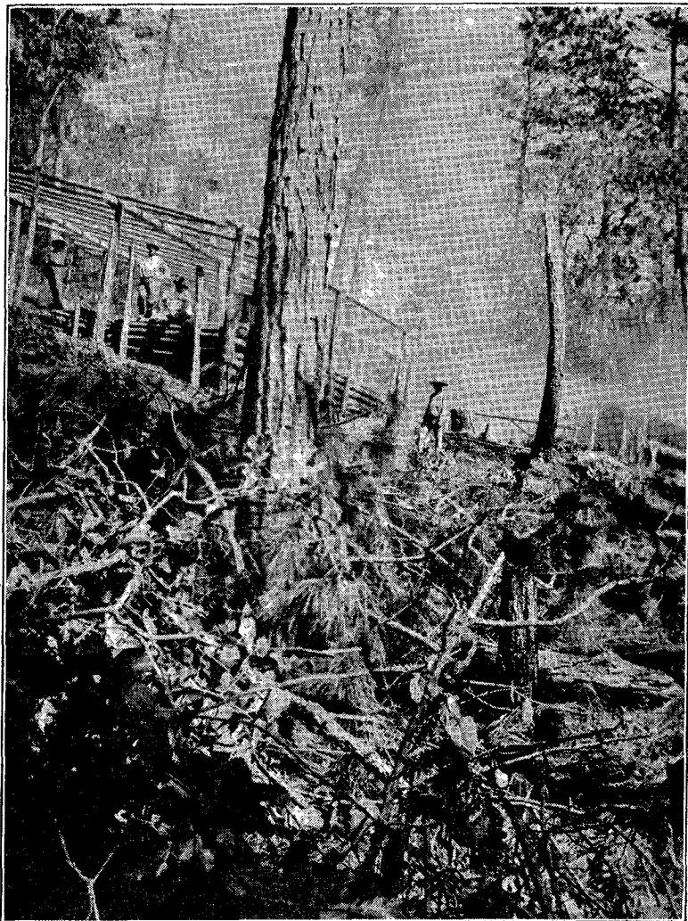
Brother and Sister Hardt and their first School Building in process of construction near Siguatepeque, Honduras
