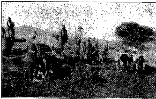
Beginning of the Training School at Spion Kop, Natal. J. I. Robison molding brick.
