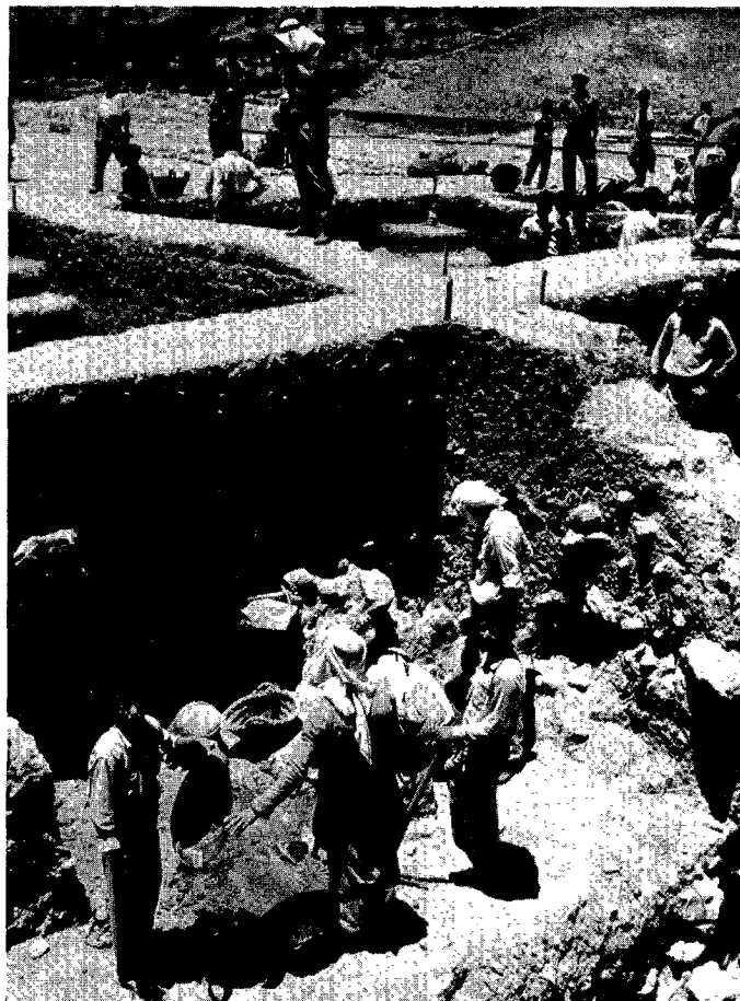
Excavating Field VII. The earth walls seen in the picture are left standing for control purposes and are later removed.
