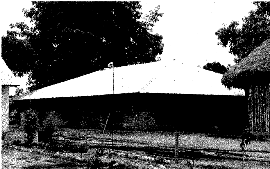
The Nevati Clinic as it neared completion. This small medical facility will serve the Campa and Amuesha Indians of the Peruvian jungle. No other medical help is available.
