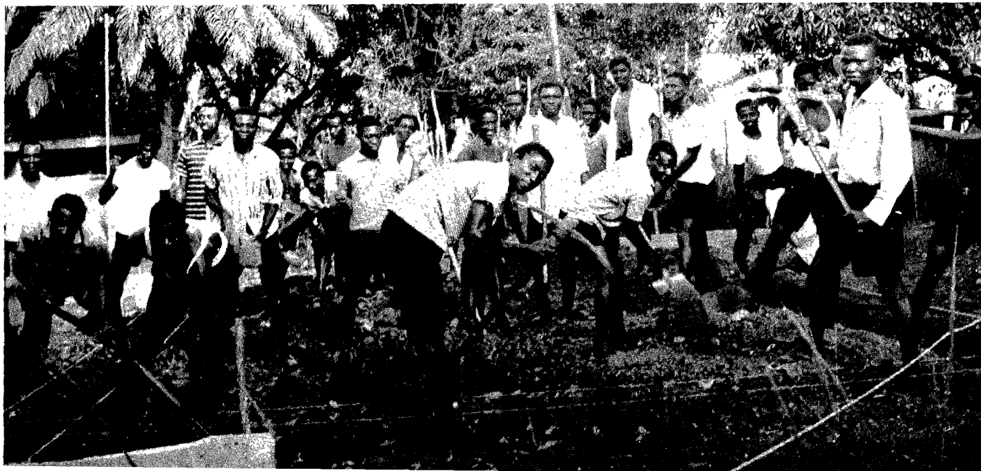
Students at Bekwai Training College digging the foundation for a new faculty home. Students carry on evangelism in nearby villages.
