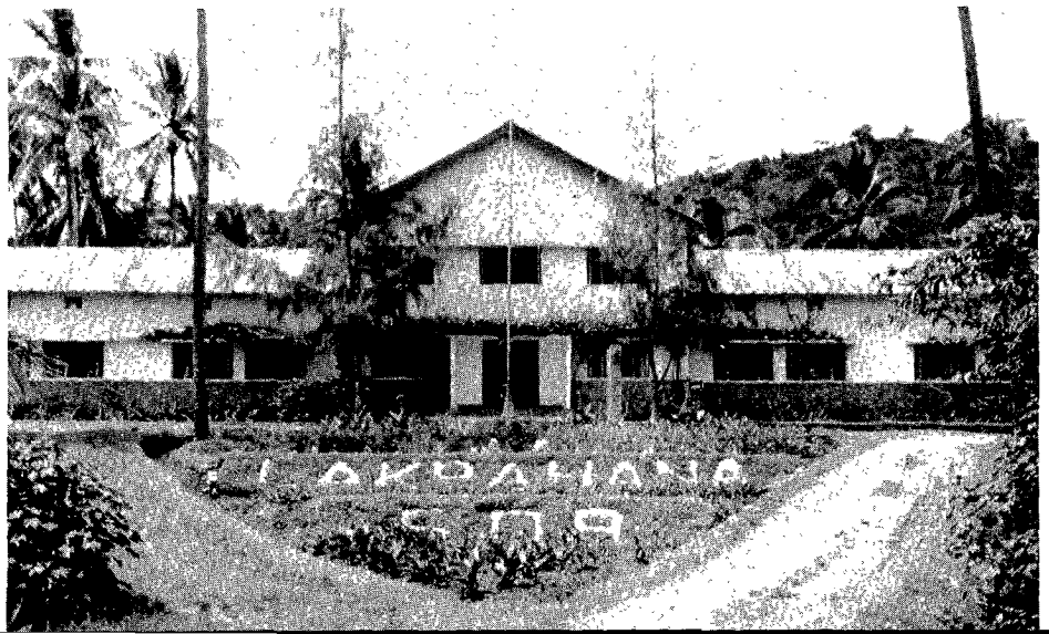
The administration building at the Lakpahana Training Institute in Ceylon.
