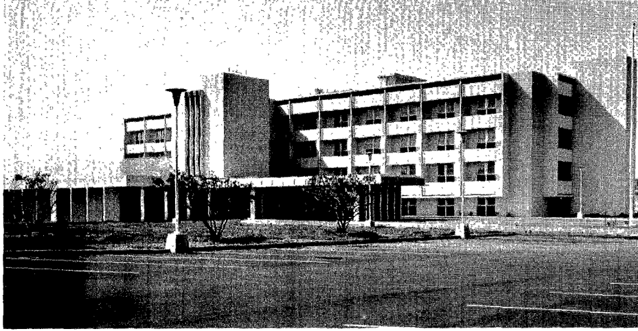
The new Paradise Valley Hospital in southeastern California provides more than 138,000 square feet of usable space. The five-story steel-and-concrete structure is located on an 11-acre site. One story cannot be seen in this front view.
