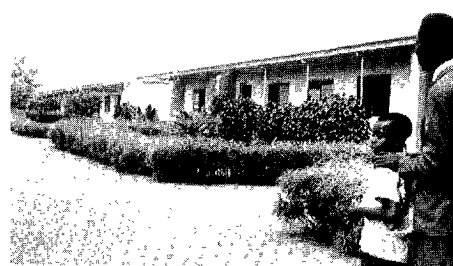
The classroom block of the Ede Secondary School, located at Ede, Nigeria, West Africa.
