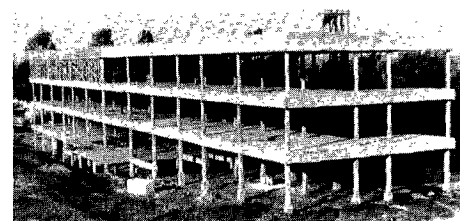
Dormitory construction for student nurses is under way at the River Plate Sanitarium.
