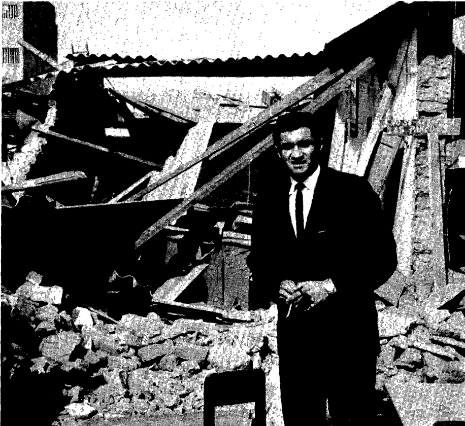
Guillermo Bonilla, SAWS public relations worker, stands in front of the rubble of the church and school in Chimbote. The hand-lettered sign says, "Don't lean on the walls."
