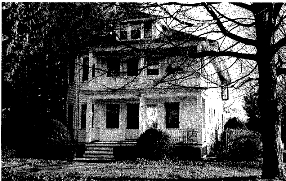
This building, on Bolton Road, South Lancaster, Massachusetts, was Southern New England Conference headquarters for some 22 years. It also contained the Book and Bible House, and provided living quarters for a number of conference presidents.
