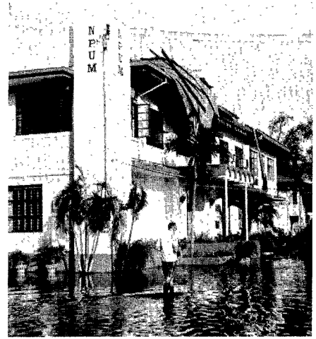
The North Philippines Union office roof was extensively damaged by the storm.
