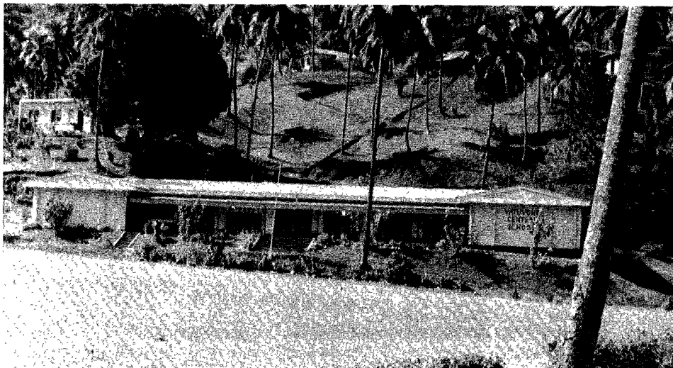
The Vatuvonu Central School is situated on Buca Bay on the island of Vanua Levu.
