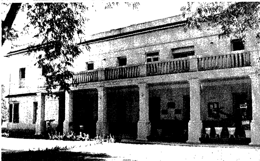
River Plate Sanitarium and Hospital in Argentina opened in 1908 and has become the South American Division's largest medical institution. The top picture shows the building as it was originally constructed; the bottom picture shows it from another corner as it is now.
