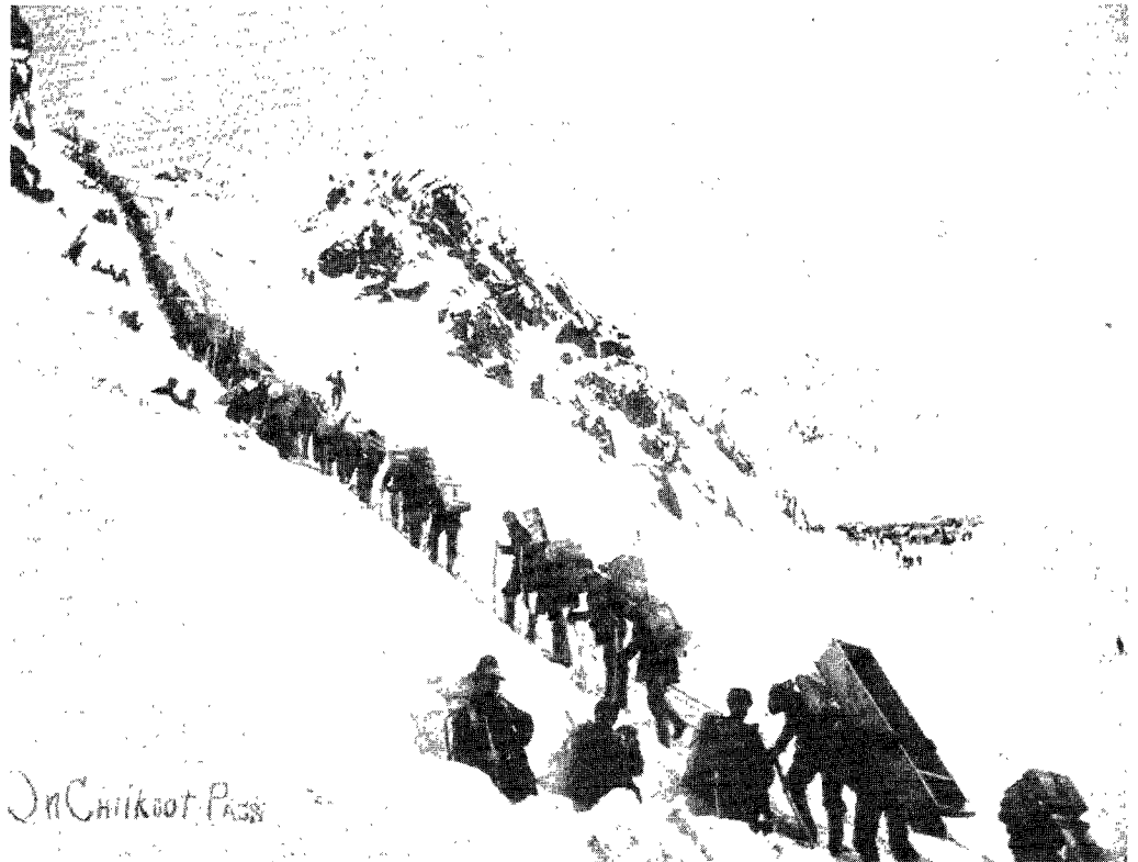
During the gold rush in the late 1890's, thousands of men trudged over dangerous Chilkoot crossing to get to Dawson City. All that mattered to them was the yellow metal that lay along the bottom of the Yukon streams.
