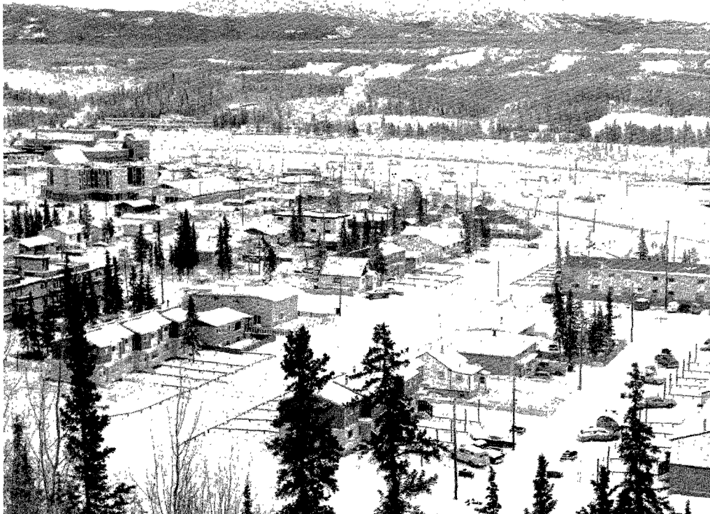
Maranatha Flights International volunteers plan to build a church in Whitehorse in June, as well as to visit people in the community. Six Union College students will spend the summer visiting and giving Bible studies.
