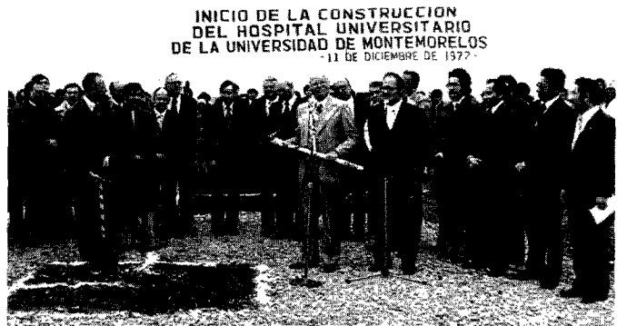
December 11 was groundbreaking for the university's medical center.
