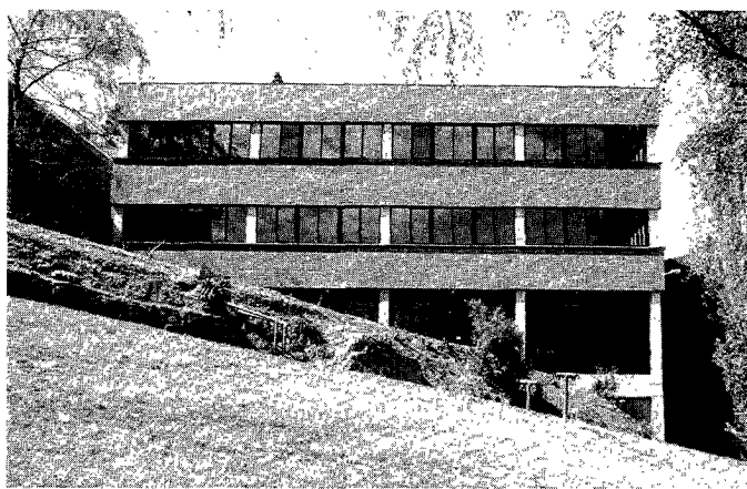
The health-education wing at the Warburton Health Care Centre contains a 20-meter heated exercise pool, gymnasium and recreation equipment, offices, counseling rooms, and other health-education facilities.
