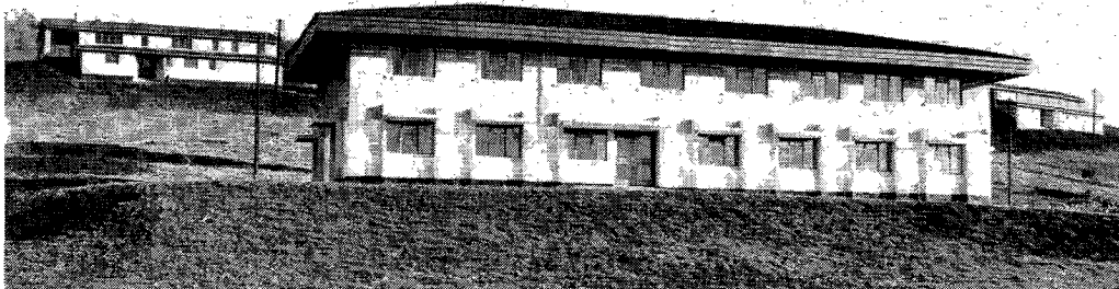
The new Tanzania Union office has wide eaves that give shade from the sun. In the background are staff houses.
