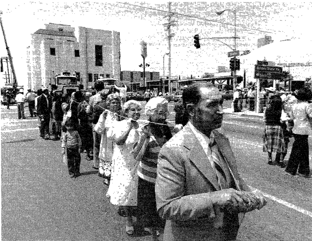
Members of the Los Angeles Spanish-American church hold cords attached to their building as it is being moved.
