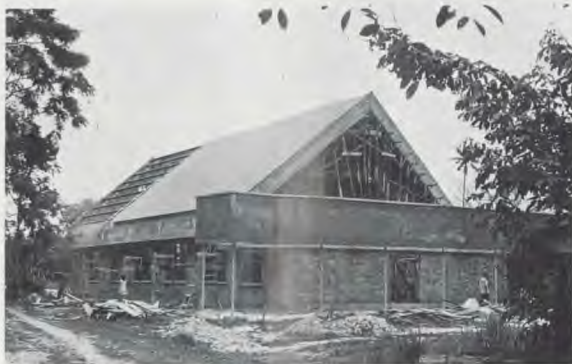
Now under construction in Ipoh is this beautiful Adventist church.
