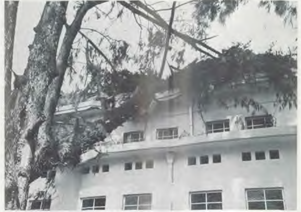
The Balestier Church was damaged when a violent wind storm uprooted this tree.
