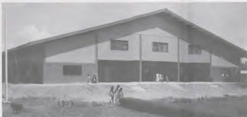
New Goshen Auditorium with a seating capacity of 3000.
