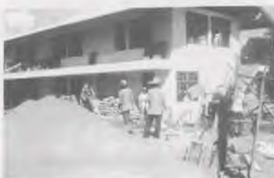
The finished product beginning to shape up.
