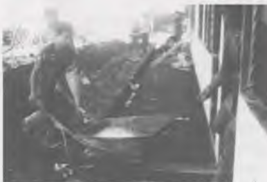
Pouring the cement floor, one wheelbarrow load at a time.
