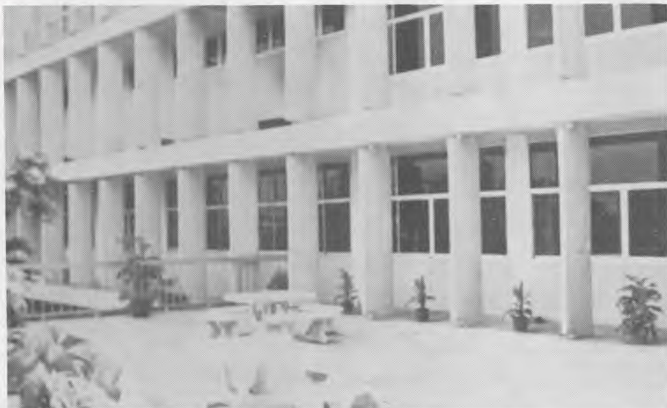
The second floor patio of the Ralph Waddell Wing lends itself beautifully to dinners and receptions since windows in the Health Education kitchen may be opened for convenient serving purposes.
