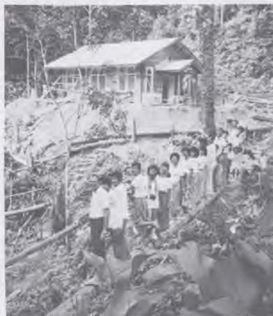
The Lightbearers cross the new long bridge leading to the church.
