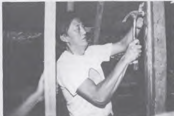
Dr./Pr. David Wong nails boards on the church building.
