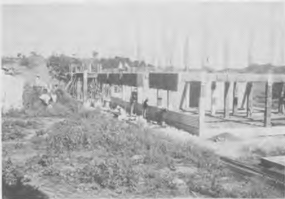
Girl's dormitory going up.
