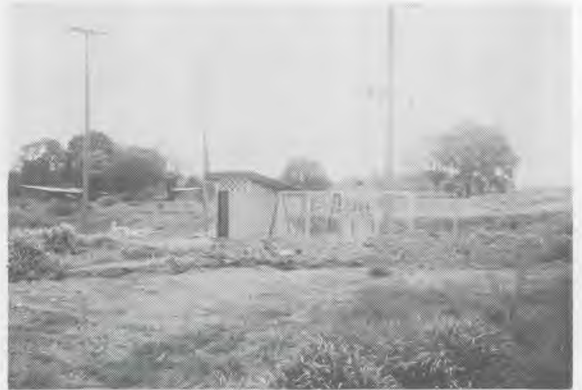
High voltage electricity at Muak Lek; the campus first received electricity on August 7, 1989.
