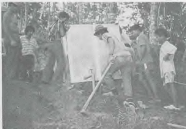
Villagers help set a water storage tank in place.
